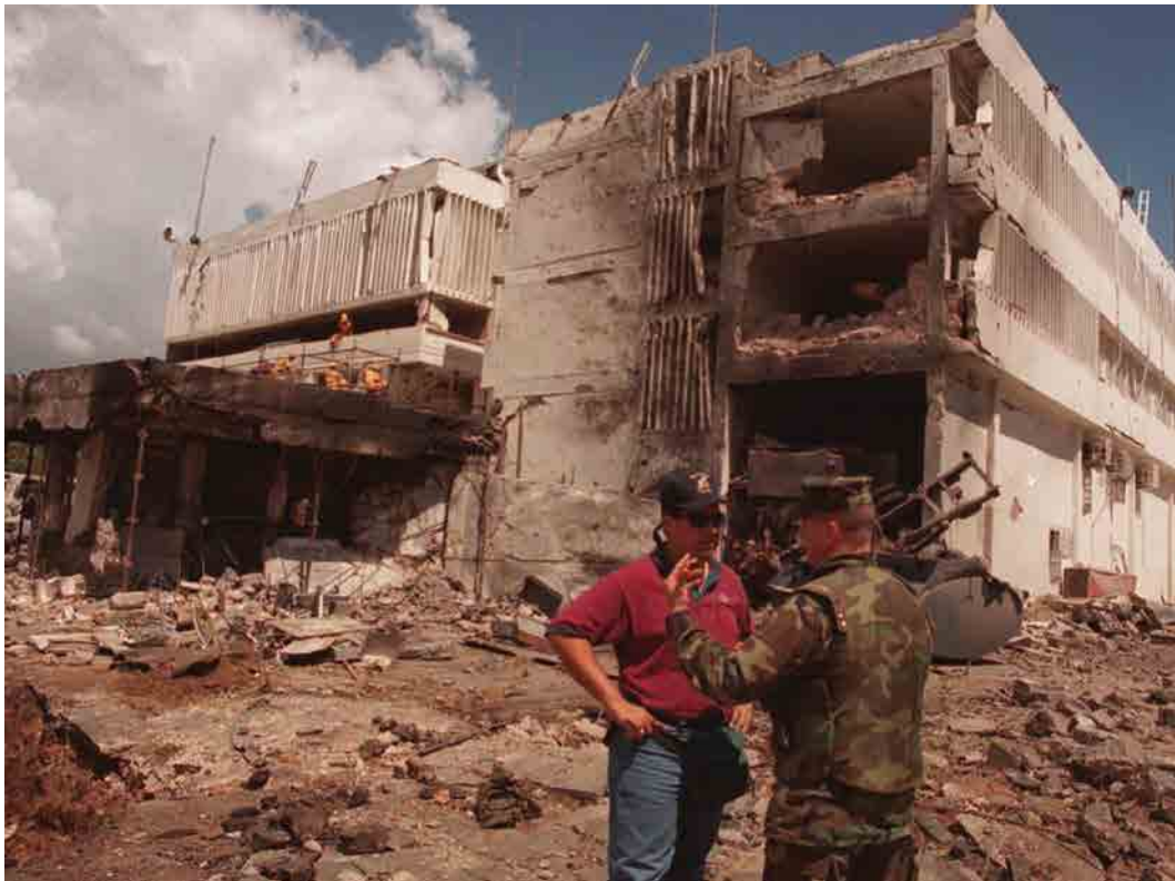
The U.S. Embassy in Dar es Salaam, Tanzania, in the aftermath of the August 7, 1998, al-Qaeda suicide bombing.
